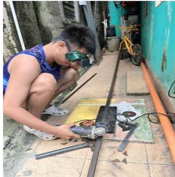
Fig. 2. Cutting and preparation of the metal frame members using an angle grinder.
