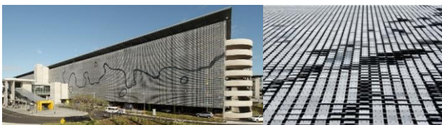
Fig. 4. Brisbane Airport Car Park and the aluminum panels used in the facade [15]
