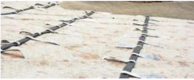
Fig. 6. Sand Blanket Leveling Above Installed PVD [30]
